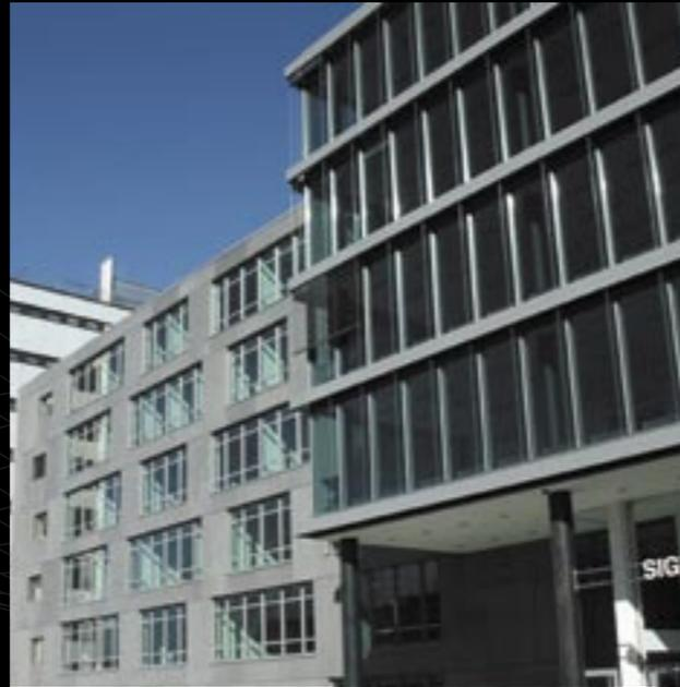
The first big project in which glassfibre-concrete was applied in the German façade-cladding-sector was produced by Fydro in Dinamic CCC. The 3.000 m<sup>2</sup> façade is built from extremely large elements with dimensions up to 8 m<sup>2</sup>. The project "Haus Rheinlanddamm" in Dortmund is recognised as a milestone in the short but successful history of GRC in the German façade-cladding-industry.
